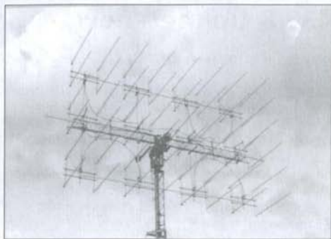
NC1I's 48 x15 rear mounted K1FO array
